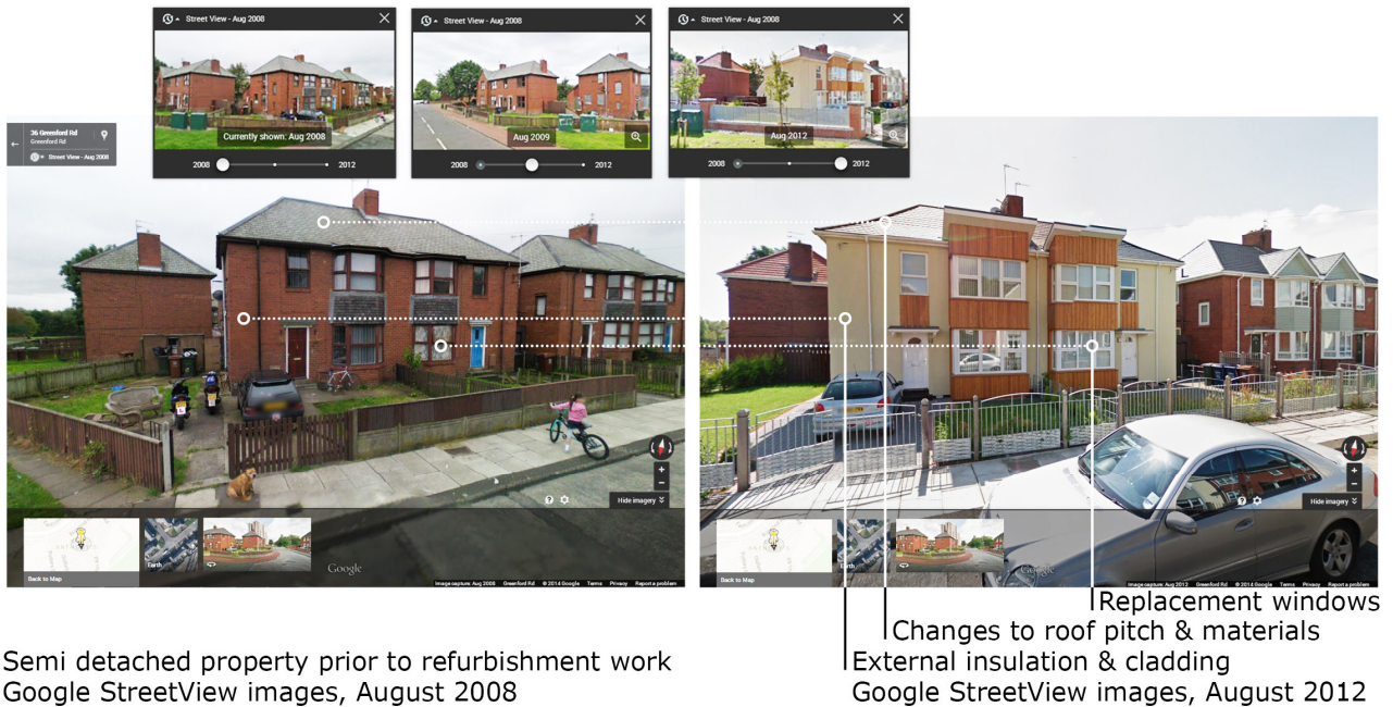
Figure 1: Potential data from historical Google StreetView for a demonstration low energy retrofit property, Newcastle upon Tyne
